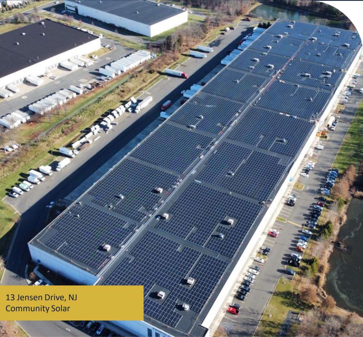
Pictured is 3.71 MW of solar under construction at 13 Jensen Dr in NJ, through a rooftop lease with Dimension Energy through 2042.<sup>1</sup> This was the first community solar project Cabot has managed. The project was awarded through the NJ Community Solar Program and is estimated to be completed in Q3 2023. The energy generated by the system will be transferred offsite and provide discounted renewable energy to low-middle income communities.
