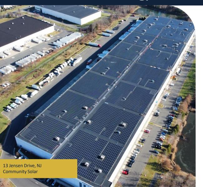
Pictured is 3.71 MW of solar under construction at 13 Jensen Dr in NJ, through a rooftop lease with Dimension Energy through 2042. This was the first community solar project Cabot has managed. The project was awarded through the NJ Community Solar Program and is estimated to be completed in Q3 2023. The energy generated by the system will be transferred offsite and provide discounted renewable energy to low-middle income communities.
